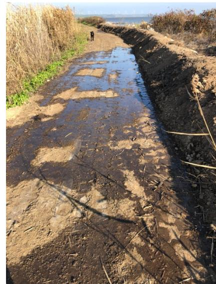
After surveying the worst spots after December 31st's high tide, I was able to determine the best places to lay 300 feet of aqua dams for protection. These dams were very effective in reducing the amount of water running over the levee on the next three high tides that occurred. However, the aquadams are only capable of holding back about 13 inches of water before they become buoyant. At the 7.13 high tide on Monday, we were
